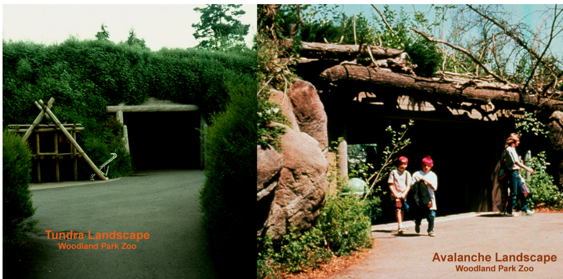
Living walls on display buildings, Northern Trails exhibit, Woodland Park Zoo. Photos: L. Sammons
